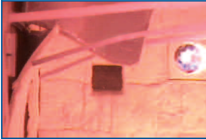
Blast Furnace superheats air and the integrity of vault remains intact as Gypsum board peels away from exterior walls.
